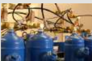
Nitrogen Purging & Pigging
